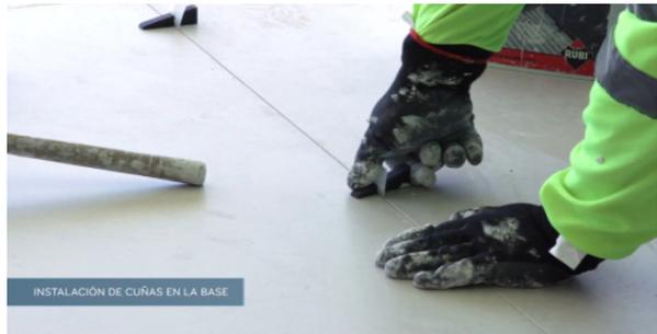
4) The Rubi Tile Levelling kit or wedges should be used for large format pieces.
