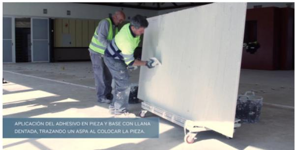
2) Combing the adhesive over the support with an appropriately sized spatula ensures the correct thickness and proper distribution over the surface, including edges.
