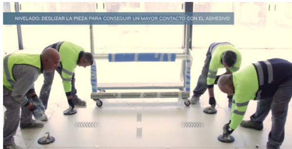
5) For the final adjustment, use movements like the ones shown in the photograph, rather than "hammering".
